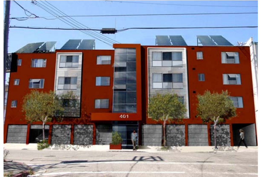
410 Fairmont, Oakland, CA - Renovation of existing apartment building for 31 new permanently affordable apartments with new community building constructed in the courtyard
