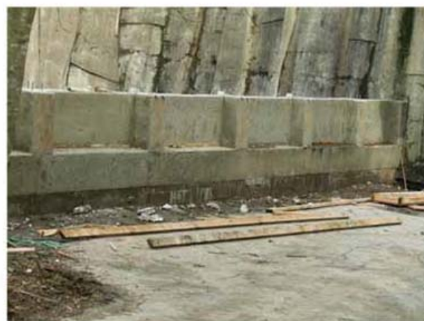
Figure 8: Stripping Forms Figure 9: Stripped Forms
