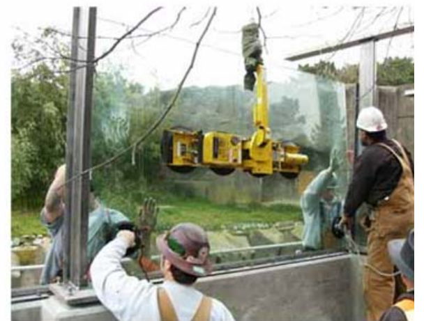
Figure 10: Formed Enclosure Figure 11: Installing Glass
