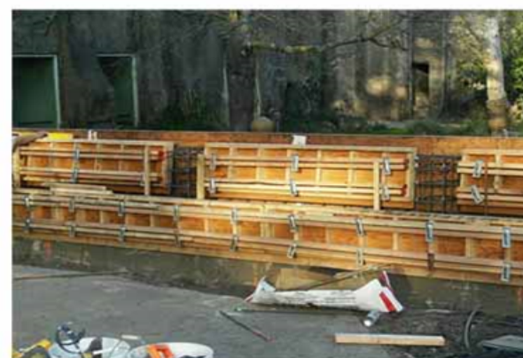
Figure 4: Inside Wall of the Tiger Grotto
