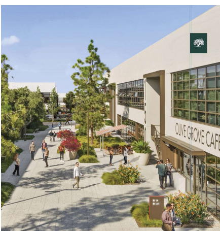
Orange County Innovation Office Park Irvine, CA 28 2-story buildings, 1.2 M SF 73 Acres LEED Gold
